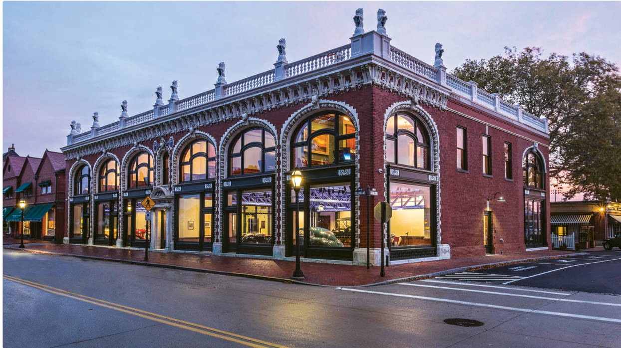
Now restored back to its original condition, the historic building once again has its rooftop balustrade and lions that were destroyed by a hurricane. New arched windows were installed and the intricate terra cotta ornamentation was restored back to its original condition. Ben Jacobsen
